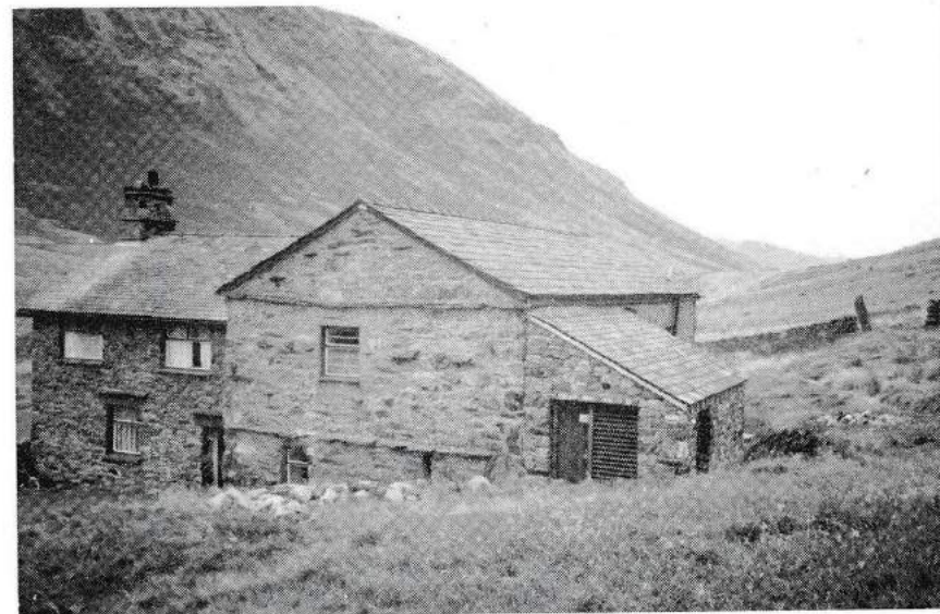
Dunmail with the new generator housing.
